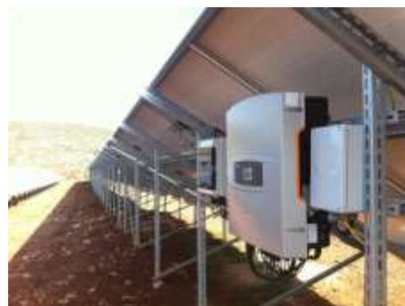
Figure 5 photovoltaic inverters generate 2kHz to 150kHz "forced emissions" into the grid
